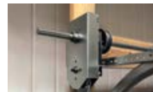
Hand chain hoist with an integral braking system provides controlled descent for sectional doors.
